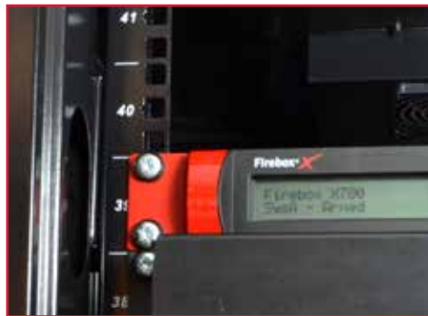
Incremental U-height markings on profiles
